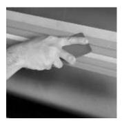
Once fully attached, use the burnishing tool to apply additional pressure to the entire PontoonGuard, ensuring the pressure sensitive adhesive is firmly attached.
